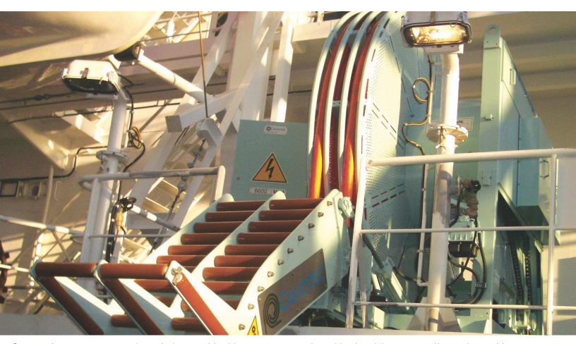
Cavotec shore power connection solutions enable ships to connect to shoreside electricity at ports all over the world.
