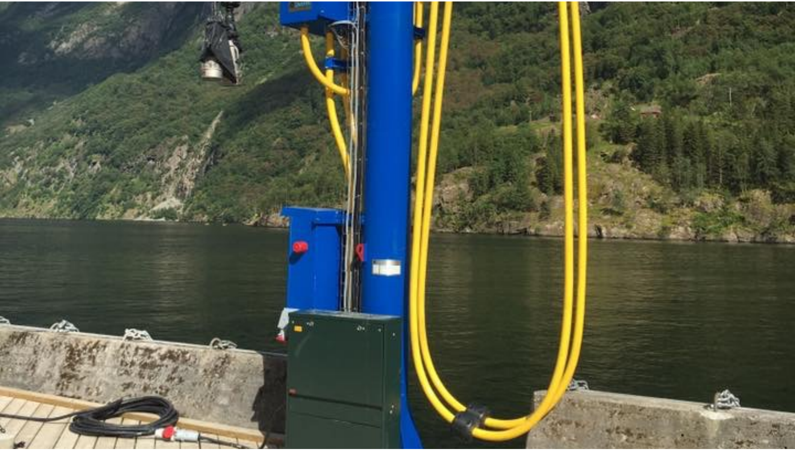
Power point: one of the two Cavotec shore power dispensers that charge the award-winning ferry.
