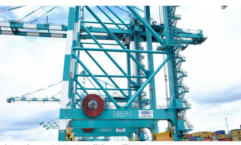
Reel power: Cavotec motorised cable reels on the ZPMC cranes at PTP in Malaysia.
